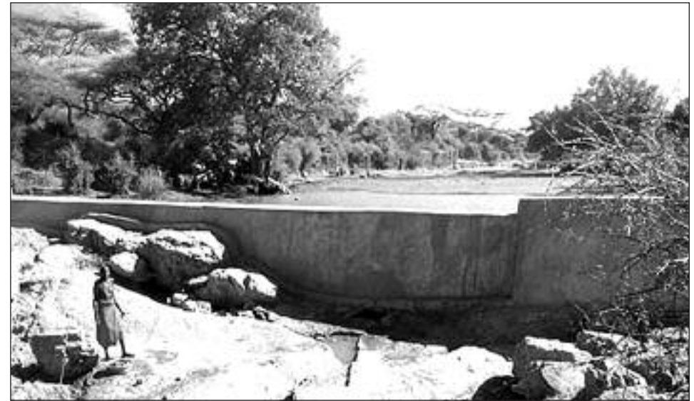
The completed dam after the rains
