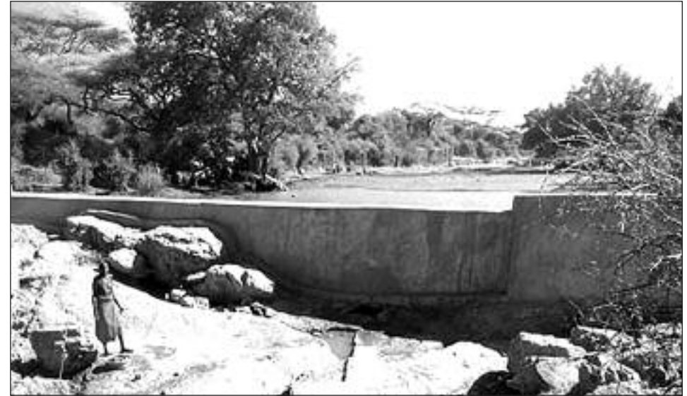
The completed dam after the rains
