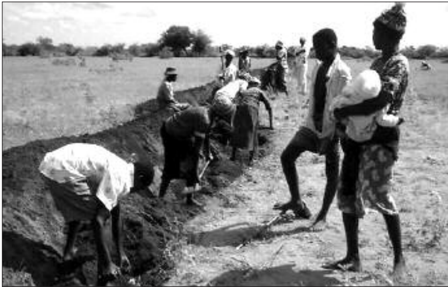
Contour ridge and infiltration pit under construction
